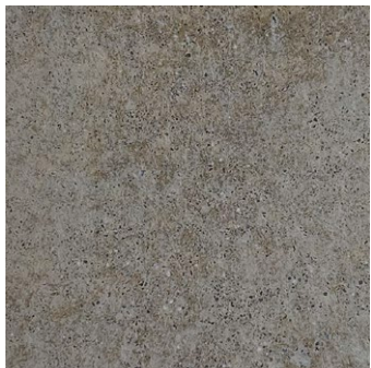
床 / Floor 磨き左官 / Polished plastering
