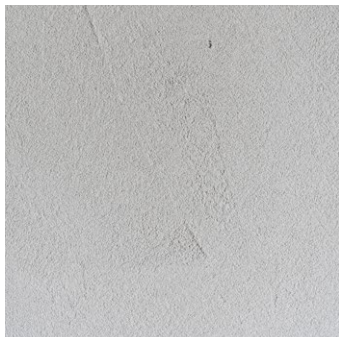
壁 / Wall 漆喰 / Lime plaster
